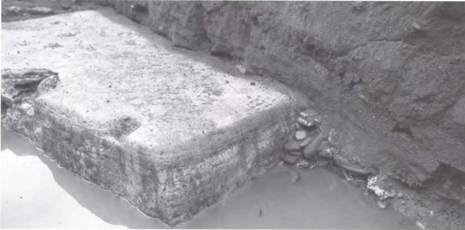
Fig. 8. Trench 21, detail of the SW corner block, with traces of weathering from wave-action.
